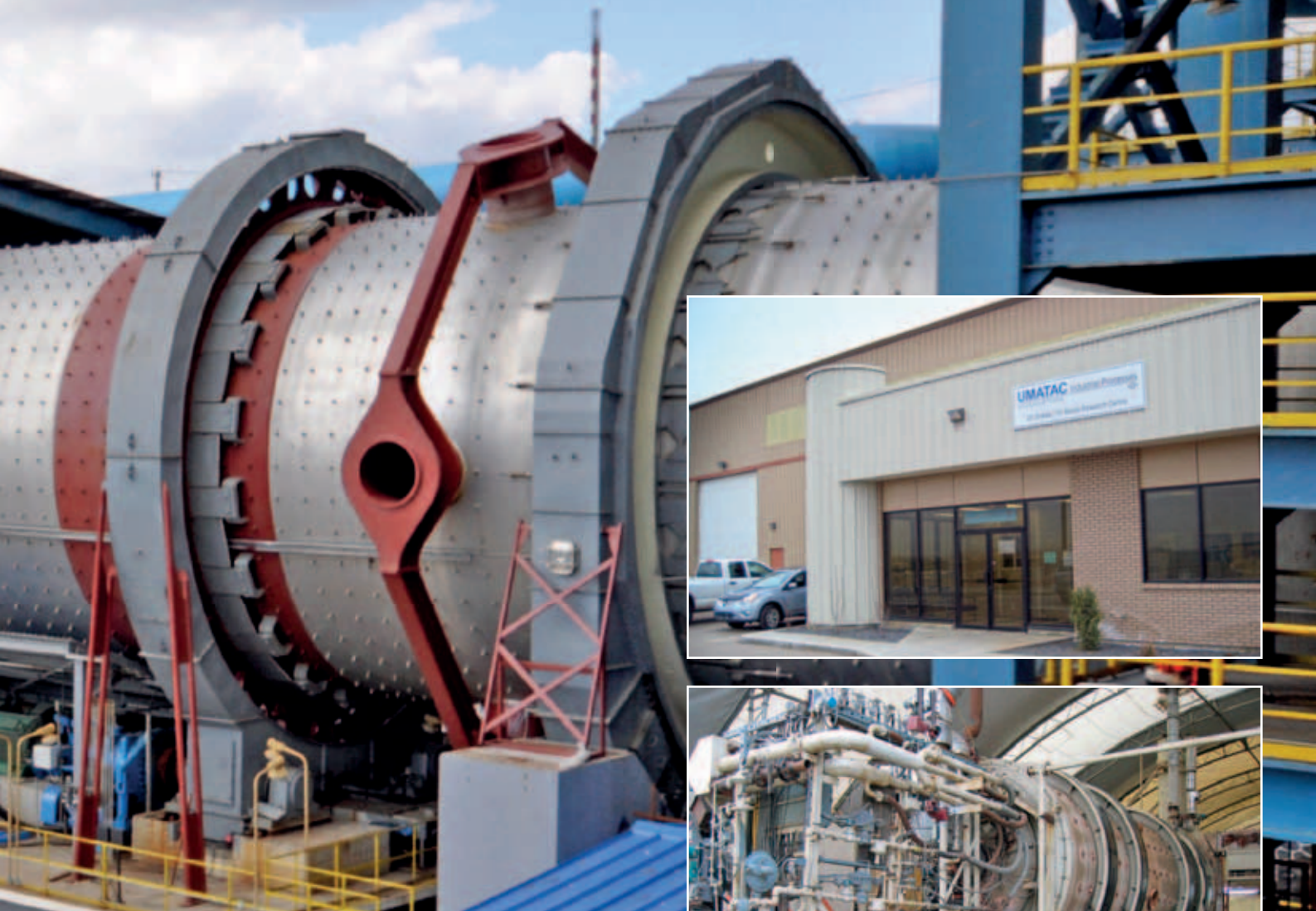
Erection of China ATP processor completed: Plant to produce more than 2,600 bpsd of light and heavy oil as well as fuel gas.
